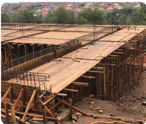
Construction under way on the Bright School campus.
